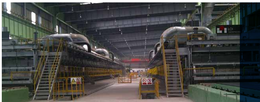
Jinan quench and temper facility
